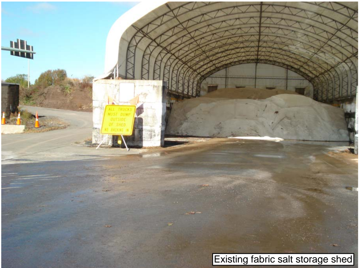
Existing storage shed to be demolished
