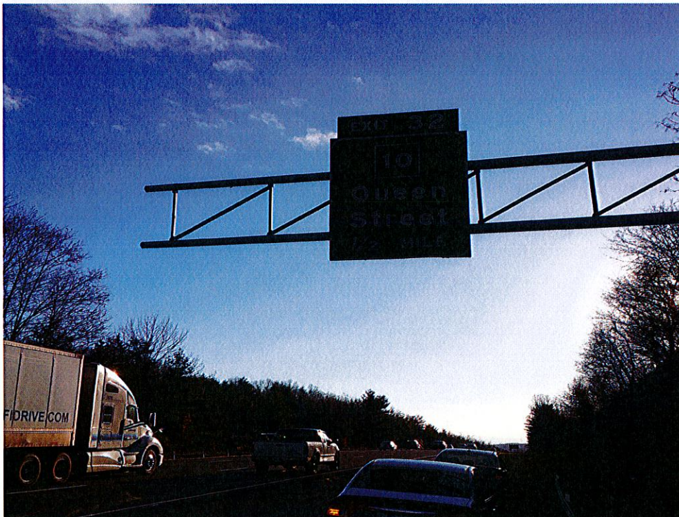
PHOTO 8 Site No. 8 – Sign Support No. 21700
