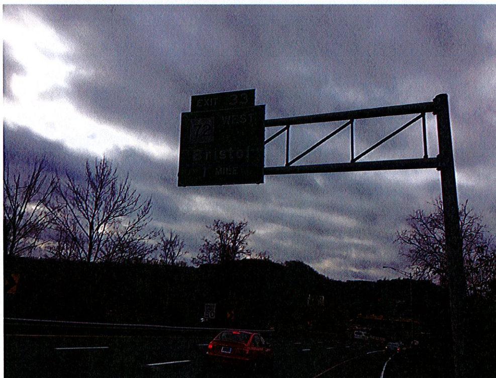
PHOTO 6 Site No. 6 – Sign Support No. 21696
