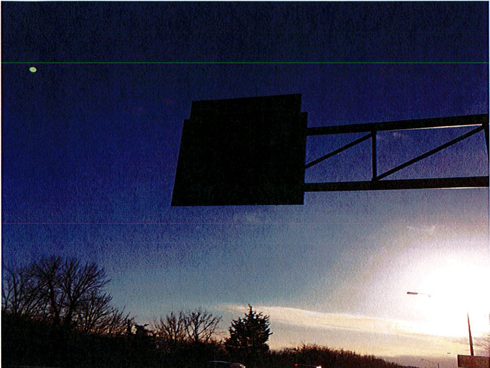
PHOTO 9 Site No. 9 – Sign Support No. 21701
