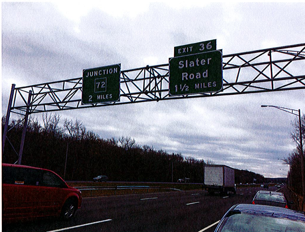
PHOTO 4 Site No. 4 – Sign Support No. 21692
