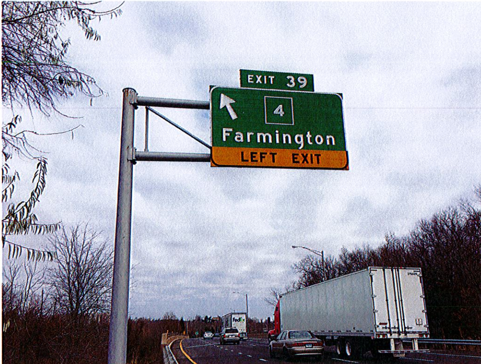
PHOTO 3 Site No. 3 – Sign Support No. 21572
