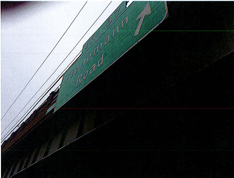
PHOTO 5 Site No. 5 – Sign Support No. 21570B
