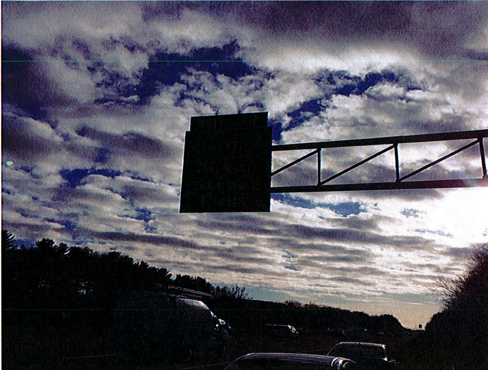
PHOTO 7 Site No. 7 – Sign Support No. 21699
