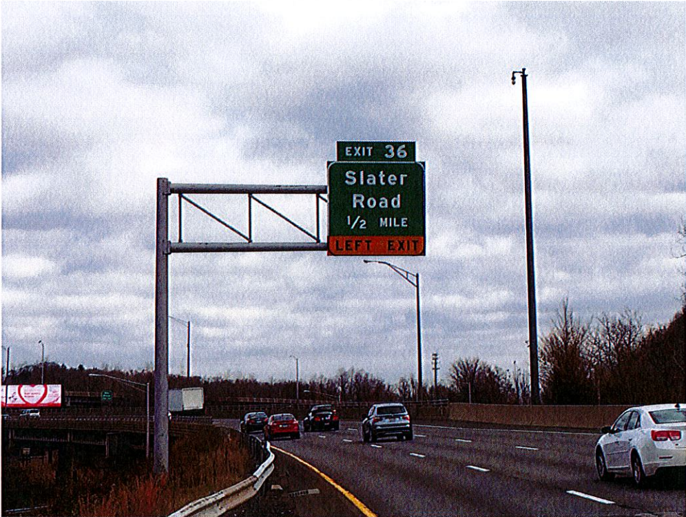
PHOTO 2 Site No. 2 – Sign Support No. 21563
