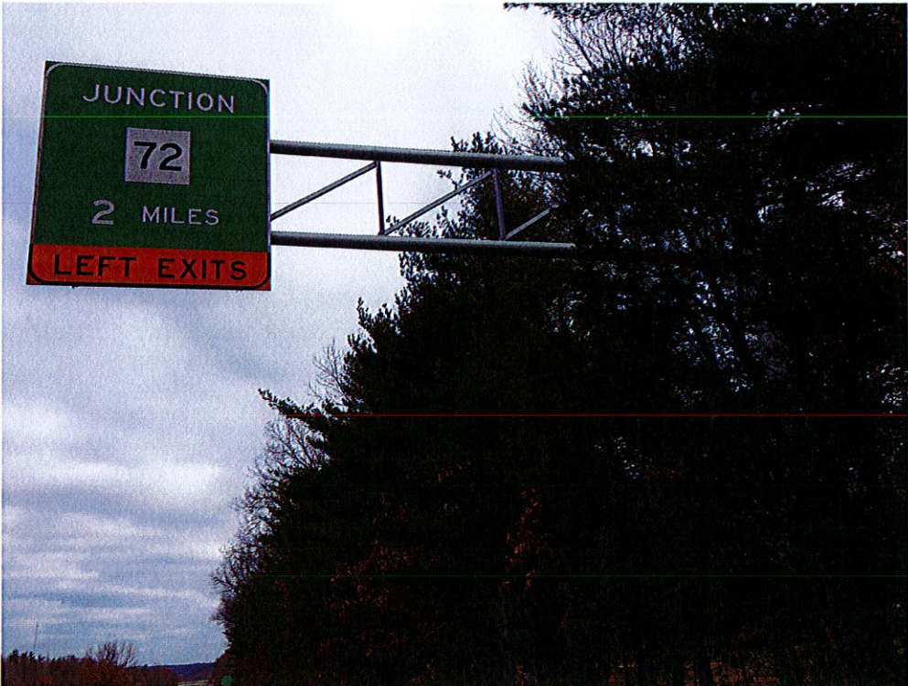
PHOTO 1 Site No. 1 – Sign Support No. 25555
