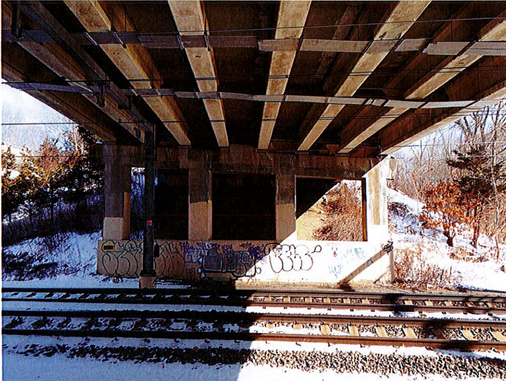
PHOTO 3 Bridge 03331 – Underside (presumed transite panels)
