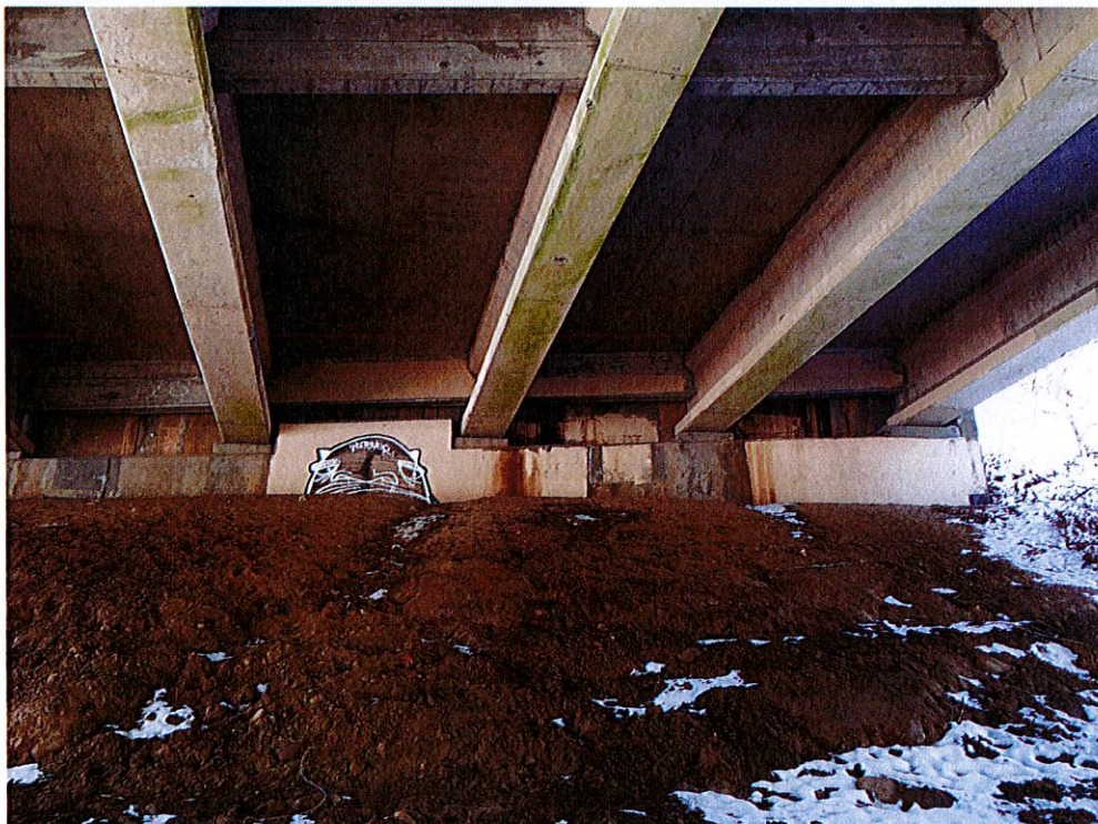
PHOTO 4 Bridge 03331 – Underside (abutment)
