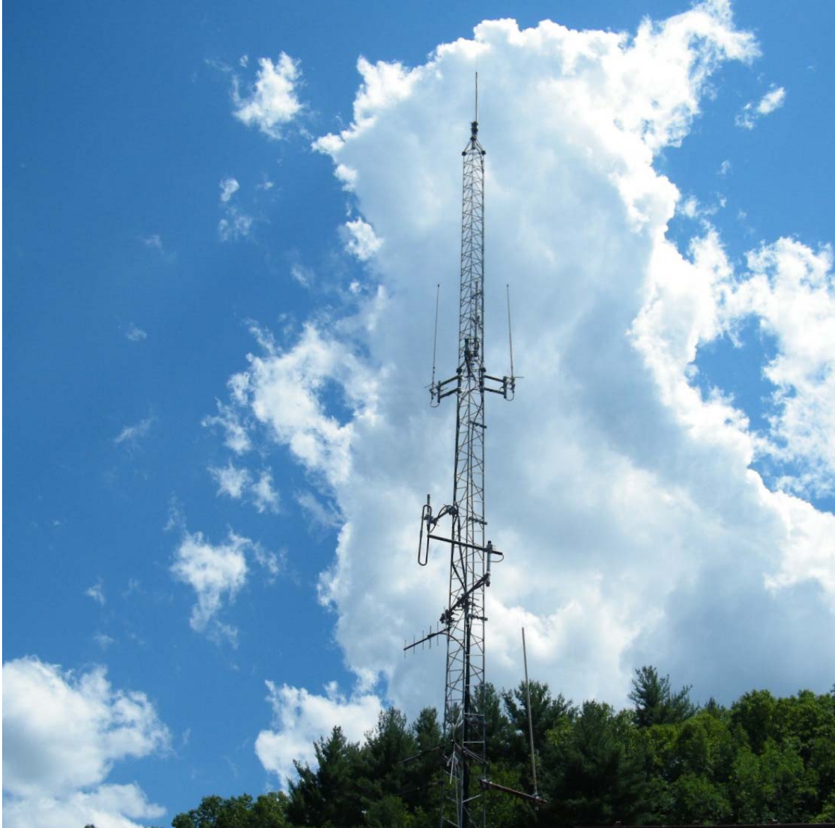
Figure B.2 – Existing Tower Middle/Top
