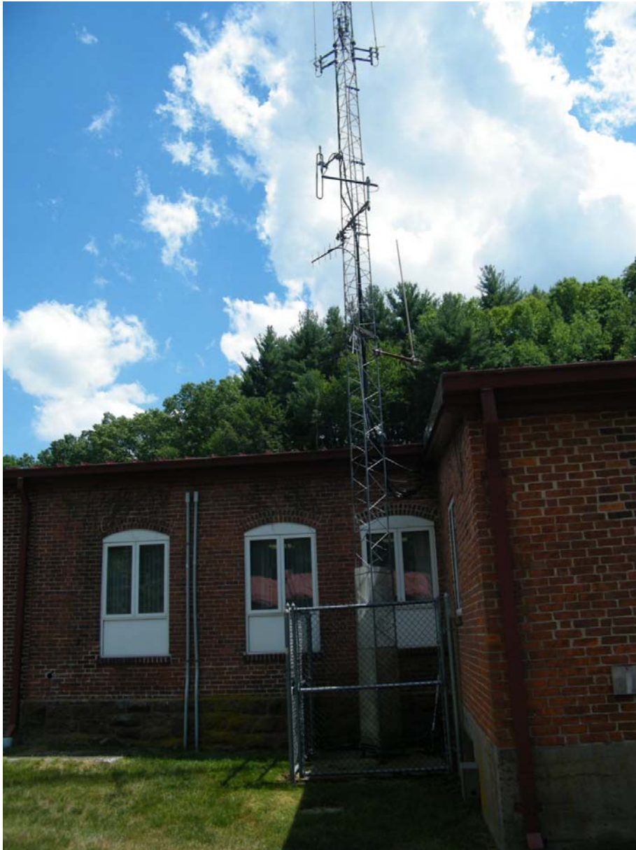
Figure B.1 – Existing Tower Base
