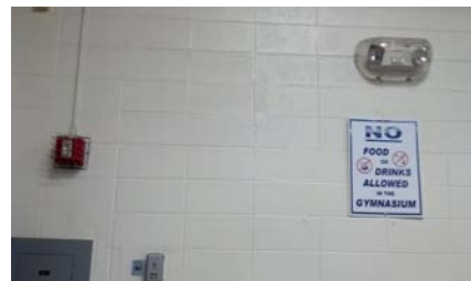
Typ. Emergency Lighting Fixture
