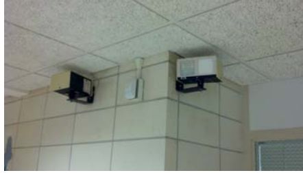
Typical Motion Detectors
