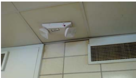
Typ. Emergency Lighting Fixture
