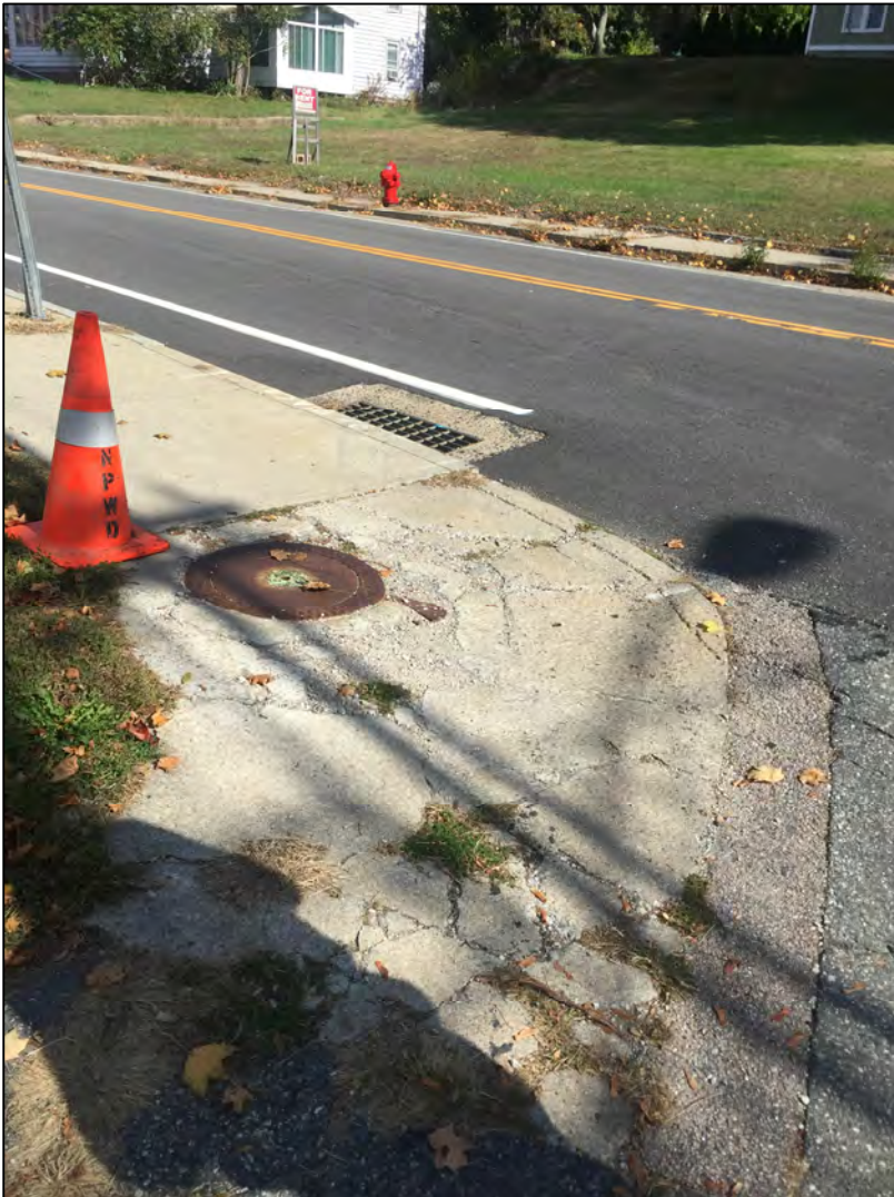
Laurel Hill Avenue (Rte 12) @ Center Street (Northwest)
