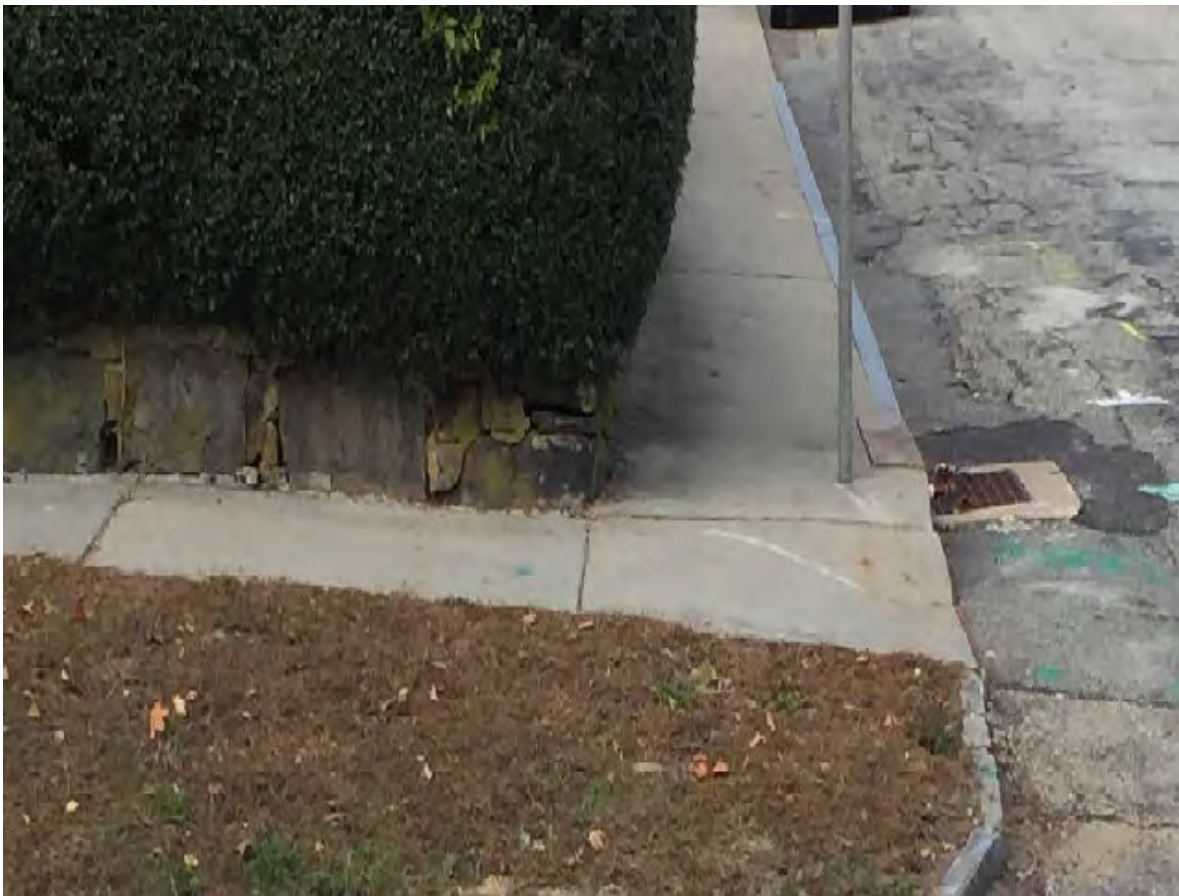
Central Ave. & Fourth St. (Southwest).
