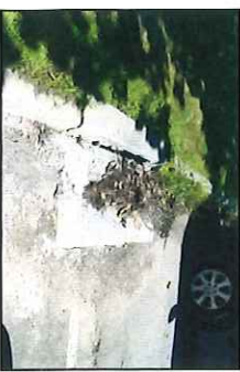
Conc. Curb at Parking Area
