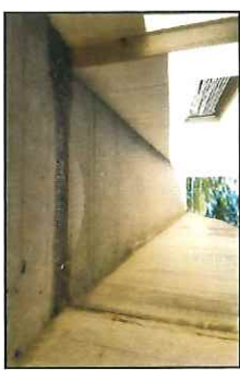
Conc. Handrails at Plaza 1
