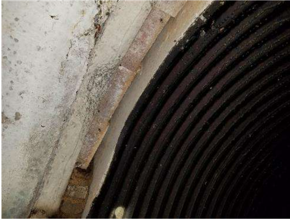
Concrete interface at east wall
