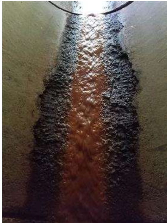
Invert of concrete pipe. Exposed rebar and spalls up to 2 1/2" deep x up to 10' long.
