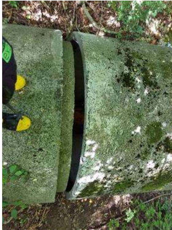
Concrete pipe separation 8-1/2" wide on outlet side
