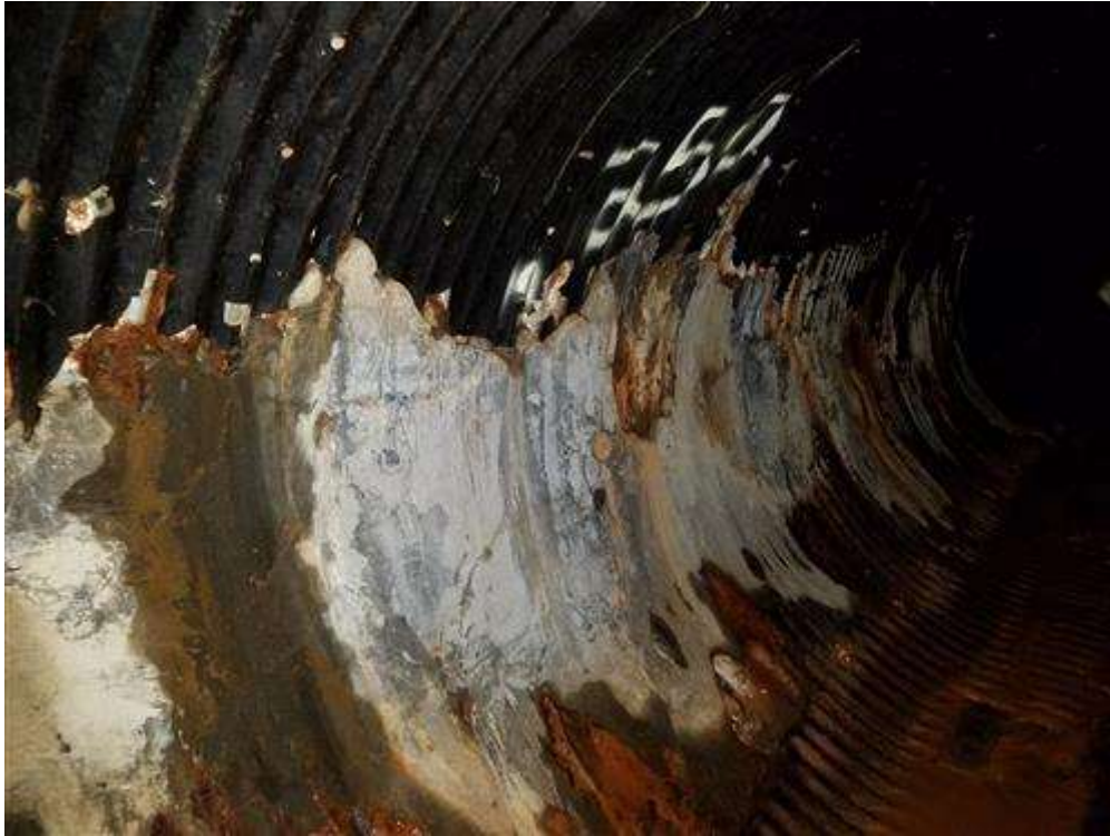
Grout repairs on west wall at 250 feet from inlet
