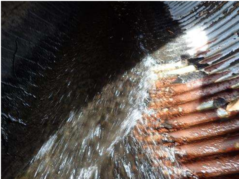
Rust on pipe along water line.
