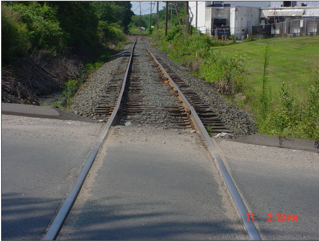
Railroad Crossing Looking North
